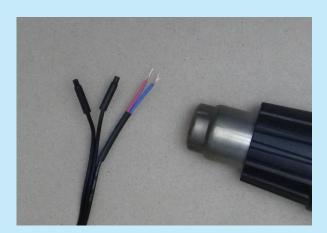
B.10 Shrink the heat-shrink tubings and end caps with the heat gun.
